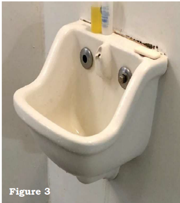
Figures 3 and 4. Detainee Cell Sink with Missing Hot Water Button (left) and a Detainee Demonstrating Filling a Drinking Cup from a Housing Unit Floor Mop Sink (right)
